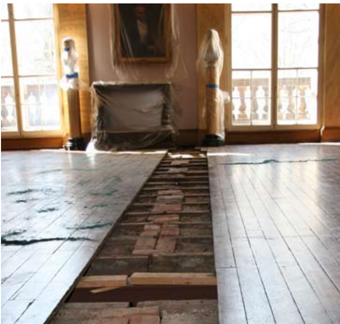
Above: Busch Room floor during south wall repairs.
